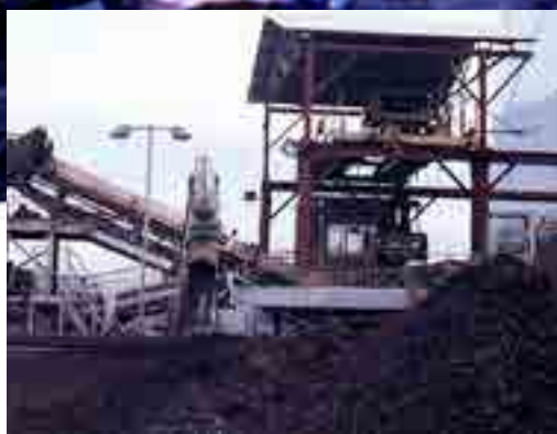
Battery breaker. (Credit: Howard Forrest)
