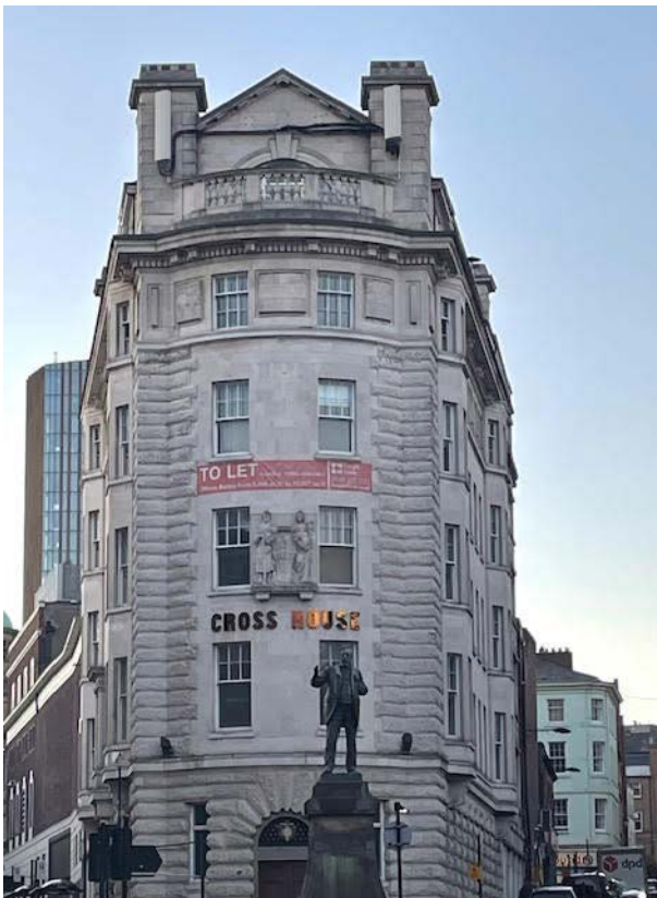
Cross House in Westgate Road (1911) was another building designed by the Cackett and Burns Dick partnership before the First World War.
