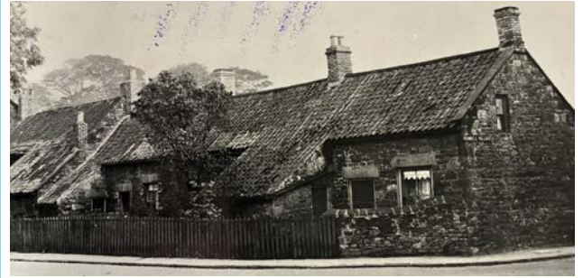
Because of the acute shortage of housing, unfit homes across the area continued to be inhabited for many years. Thirlwell's Cottages were in Old Benwell Village, a short distance from the Pendower site. They are pictured here just prior to demolition at the end of the 1930s. The Hawthorn pub was built on the site.
