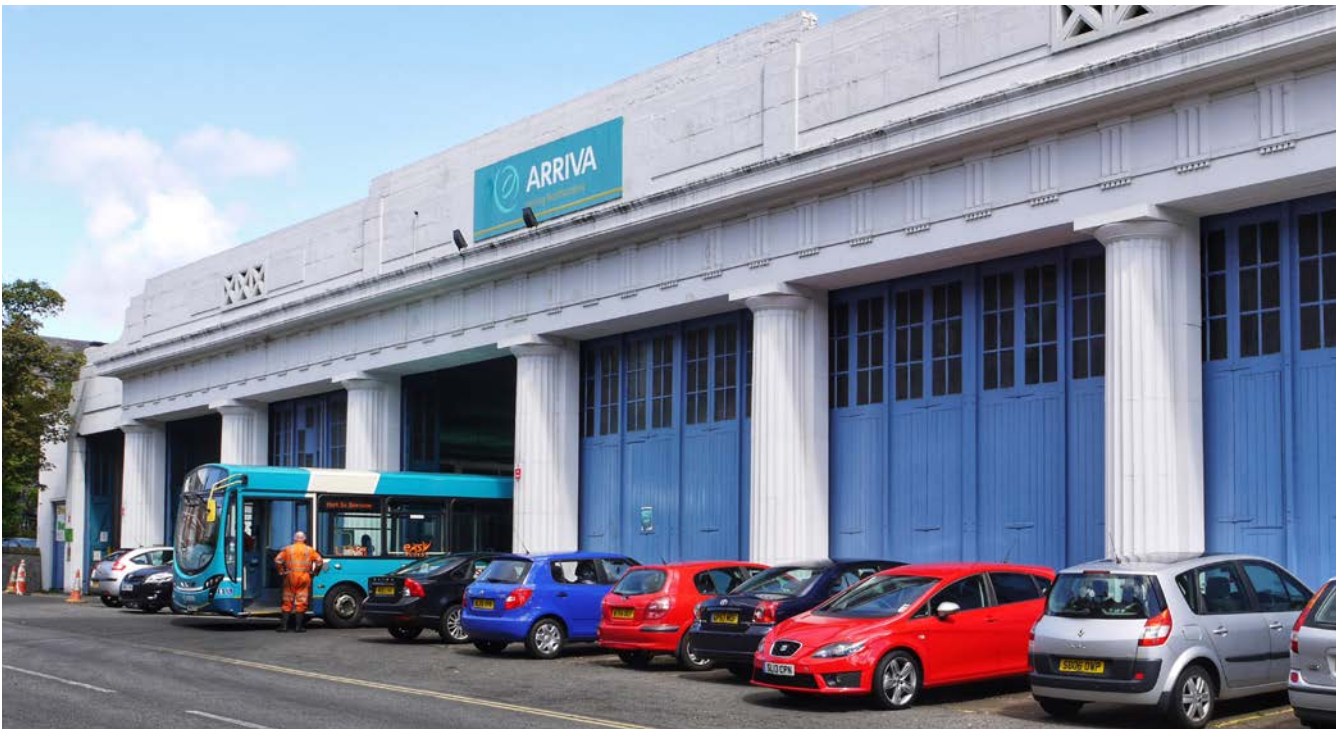
The bus depot in Portland Terrace was designed by Marshall and Tweedy for United Automobile Services. Built in 1930 in painted concrete, it has a frontage of Greek Doric columns. The building is listed but is currently vacant.
