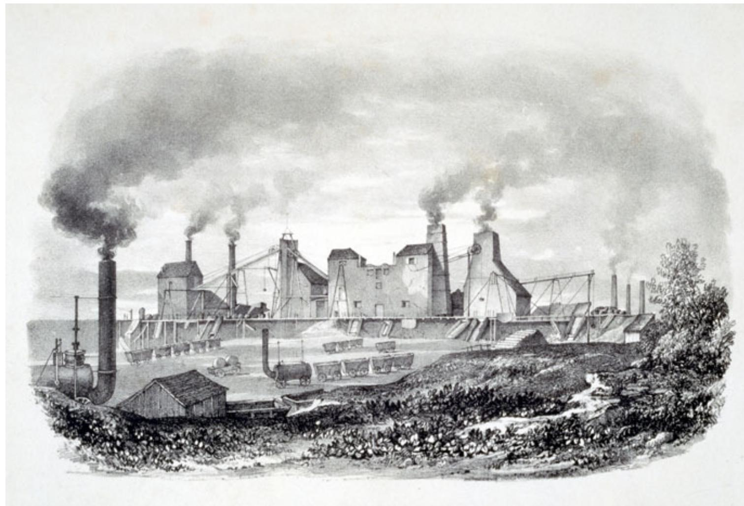
This picture shows what a colliery looked like around John Buddle's time. Can you spot the winding wheel? It moved the lifts that took men down to the tunnels underground and brought the coal up. It used steam power.
